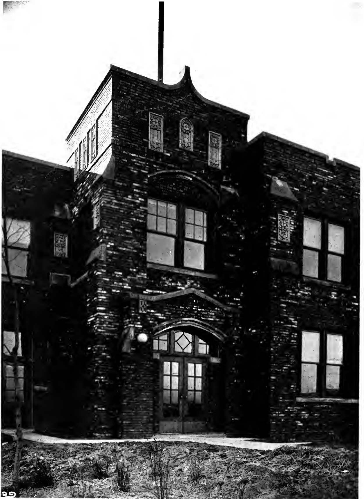
ENTRANCE DETAIL BUILDING FOR WALKER VEHICLE CO., CHICAGO, ILL. GEORGE C. NIMMONS & CO., ARCHITECTS
